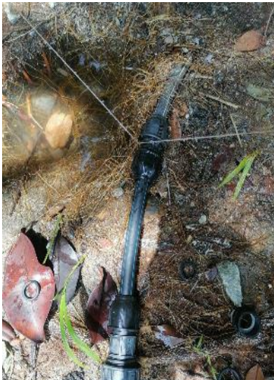
Suspected leakage
