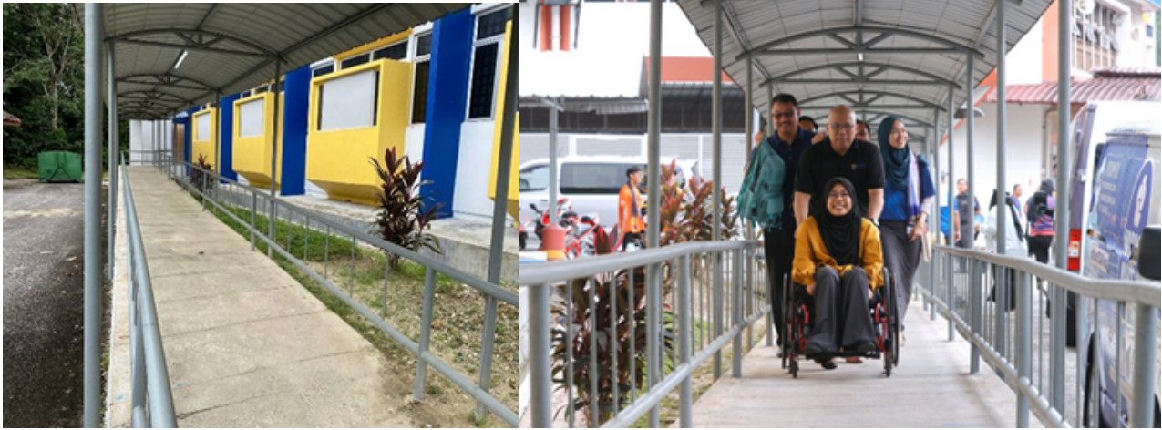
Above: A specially designed ramp in front of the student residential block, providing smooth and accessible entry for students with disabilities, ensuring safe and convenient mobility
