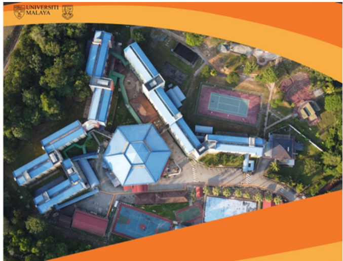
Above: Universiti Malaya's specialised residential college for students with disabilities – Kolej Kediaman Ketujuh (Za'ba)
