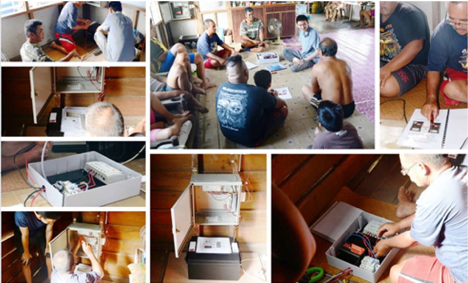
Above: UMPEDAC researchers installed a stand-alone micro solar PV inverter system donated to rural communities in Kampung Sungai Merah, Sarawak, and Long Pasia, Sabah
