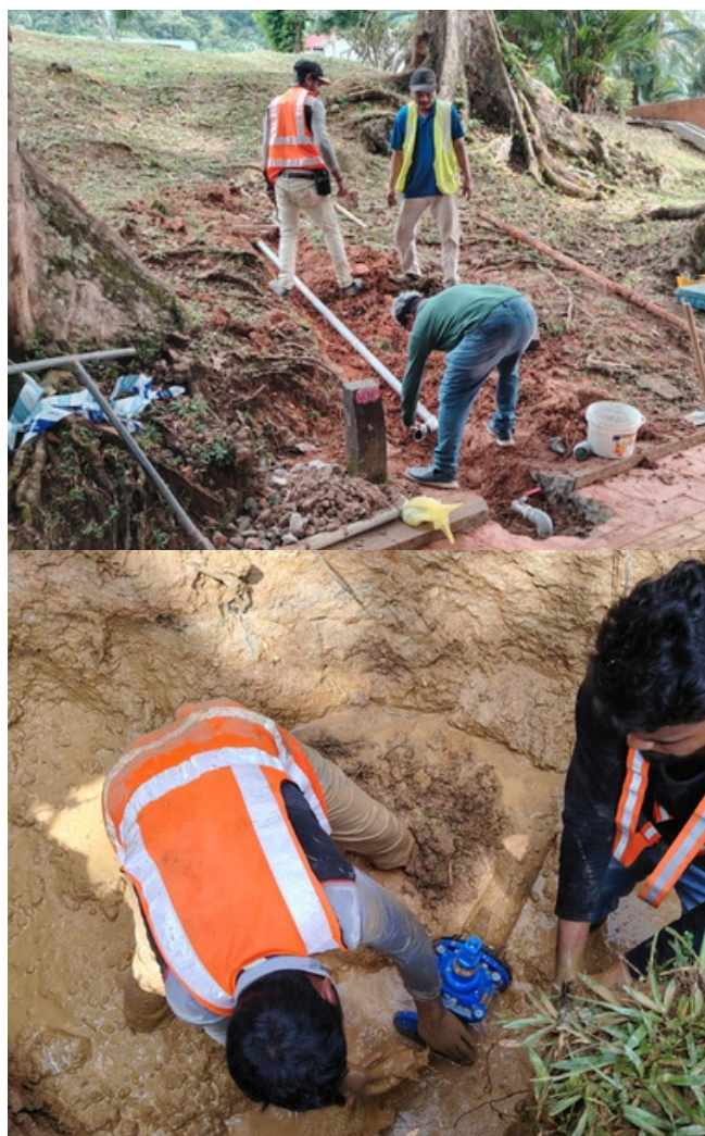
Right: Photos showing maintenance work on water pipes
